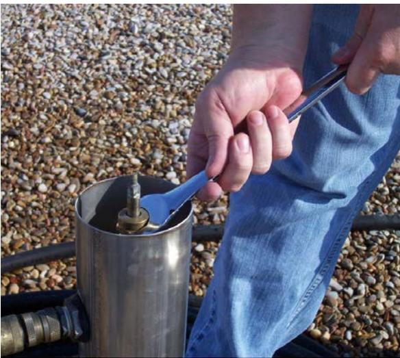
3. Remove the packing nut using a basin or other appropriate wrench.
