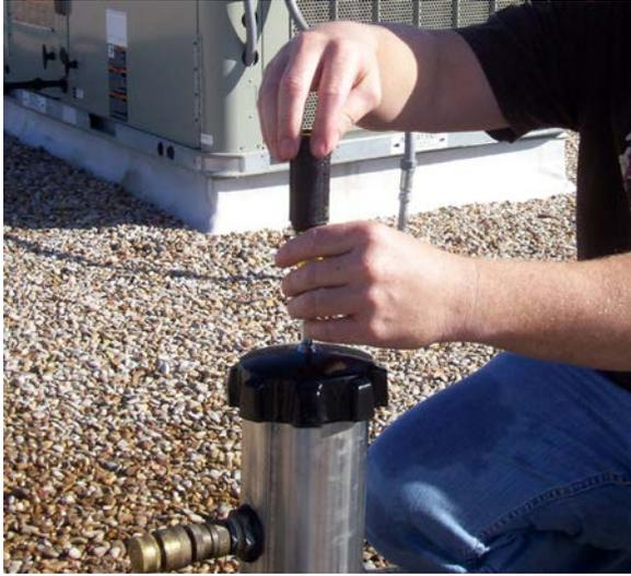
1: Remove Plastic Cap at the top of the Dome Handle.
