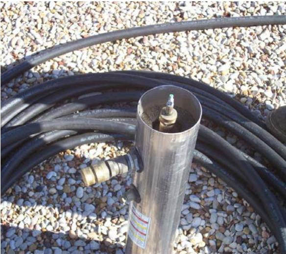
2. Loosen and remove the 1/4" lock nut and washer inside the cavity.
