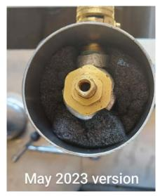
A: Remove the dome handle and look at the valve stem, bonnet and nut from the top of the hydrant.
