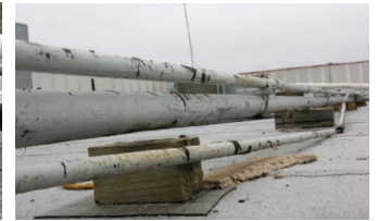
The photos above illustrate what can happen when pipes are subjected to thermal expansion without proper pipe support.
