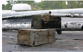
The photos above illustrate what can happen when pipes are subjected to thermal expansion without proper pipe support.
