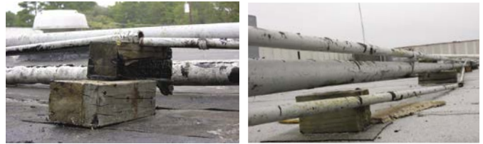
The photos above illustrate what can happen when pipes are subjected to thermal expansion without proper pipe support.
