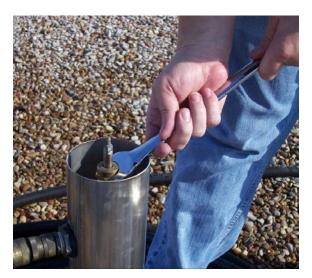
4. Remove the packing nut using a basin or other appropriate wrench.
