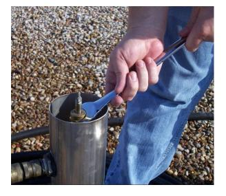
3. Remove the packing nut using a basin or other appropriate wrench.
